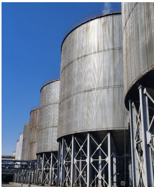
Figure 11. Upgraded clarifiers and washers.
